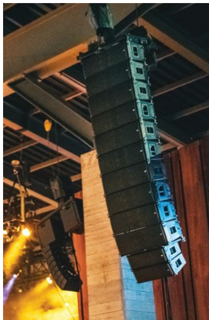
A look at one side of the VUE al-class arrays for audience and stage coverage.
